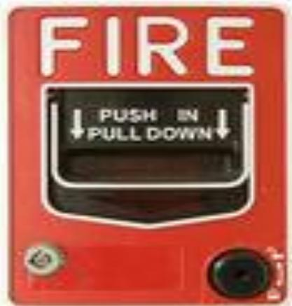
All barns owned by Fort Erie Race Track are equipped with Fire Pull stations. All fire alarms are connected to the West Gate Security Office alarm panel. All personnel living and working in the backstretch should be totally familiar with alarm and fire extinguisher locations.
